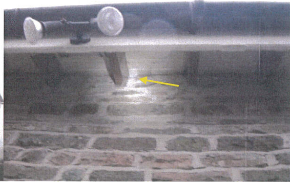
P2 Gap under west eaves
