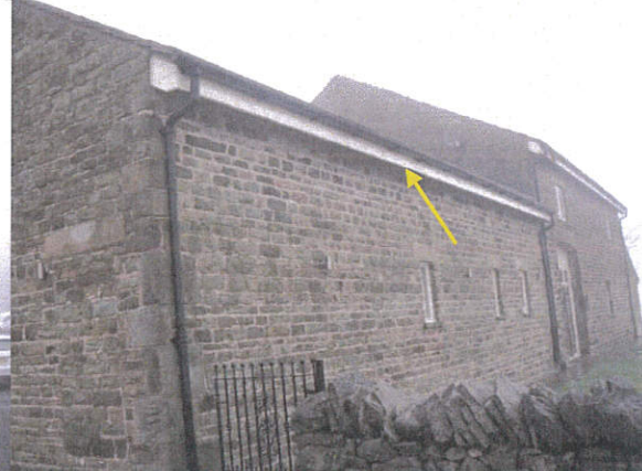
P4 East aspect, gap under eaves
