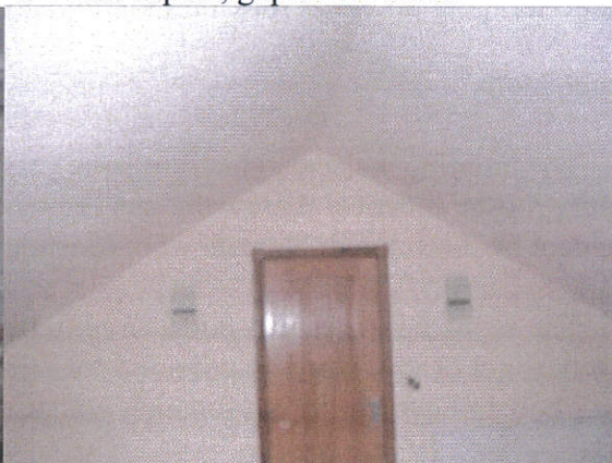
P6 Interior of Section 2, well sealed
