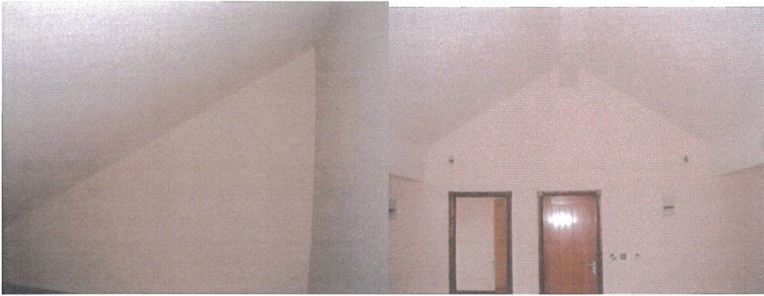
P7 Roof void – well sealed
