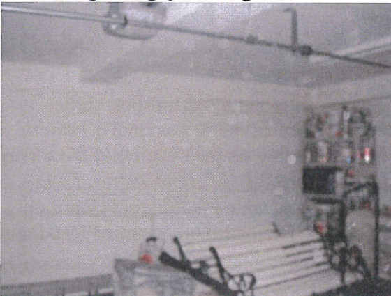
P5 Interior of garage – well sealed
